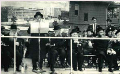
L-R: Rav Avrohom Kalmanovitch, Rav Yaakov Kaminetzky, Rav Gedalya Schorr, Rav Aharon Kotler, Rav Moshe Rivlin, Rav Moshe Chevronei, Kapichnitzer Rebbe at the groundbreaking of Yeshiva Torah Vdaath
